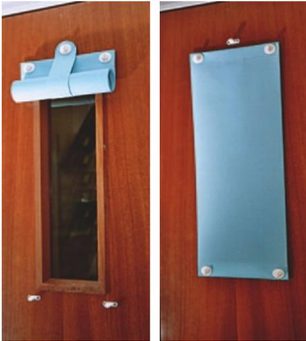
**Features:** Fabric flap with stitched hem to top and bottom, and turnbutton at each corner. Central turnbutton at bottom.
